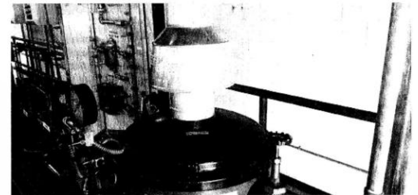
Figure 1-15 Boiler draft hood Courtesy of Camosun College
